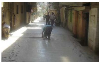
Picture (14-6) Paving roads with cement in Ezbet el-Walda
