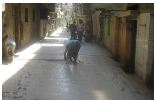
Pic. (9-9) paving roads with cement bypass
