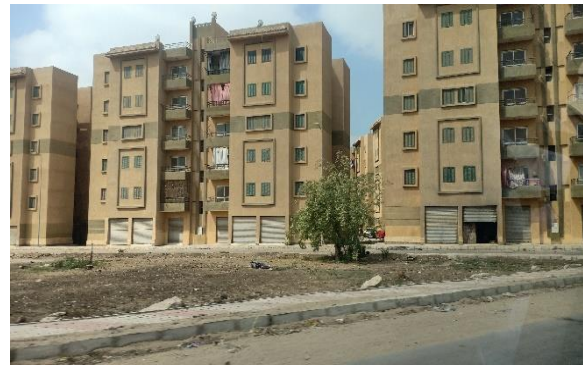
Figure 4-4: Housing projects in Arab El-Olaykat
