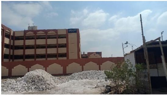
Figure 4-7 Arab El-Olaykat School Complex
