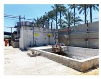
Wastewater treatment, fibre recovery and 70% recycling of treated wastewater to stock preparation and paper machine showers at Maamoura Paper, an SME.
