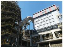
Air pollution control equipment - cooler bag filter and heat exchanger at Amreyah Cimpor Cement.
