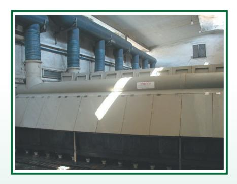
Extraction and Treatment of Fugitive Sulphuric Acid Fumes of the Battery Factory
