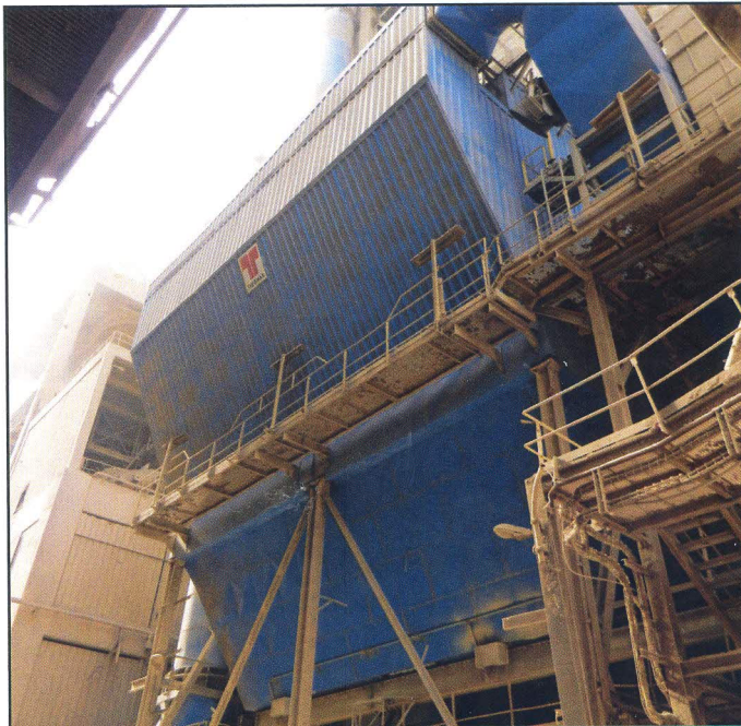
New by-pass bag filter, Line 8
