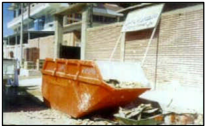
3m 3 Container Placed Outside the Tile Factory for Storage of High Density Waste
