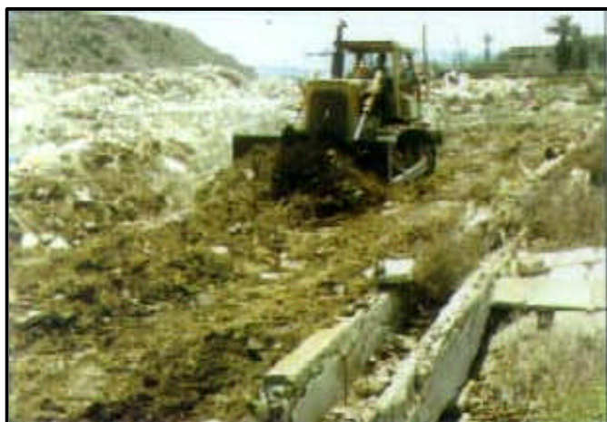
Preparing New Waste Cells and Removing Cover Materials
