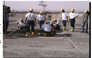
Fig. (9.6) Road pavement
