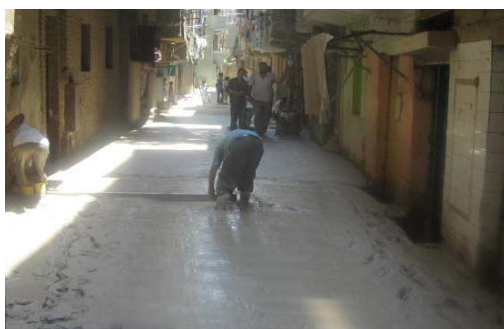
Pic. (9-9) paving roads with cement bypass
