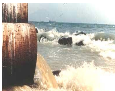
Picture (6-6) Direct Discharge into The Sea
