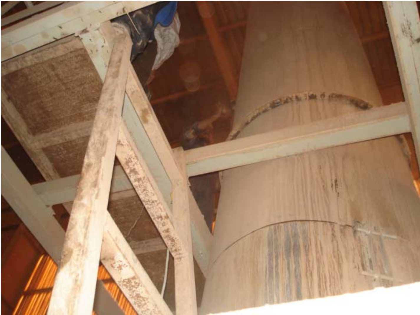
Overall view of the chimney inside the facility of ceramic corporation (planet 4)
