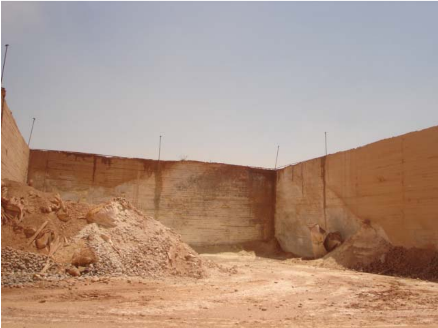
Collected suspended solids storage
