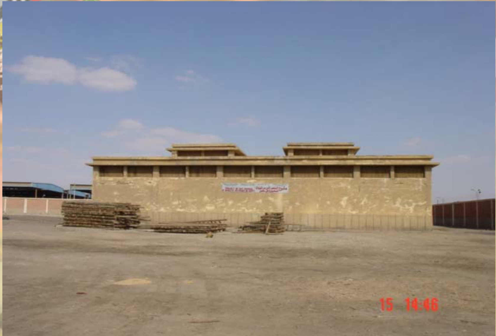
The Obsolete Pesticides Storage in El Saff
