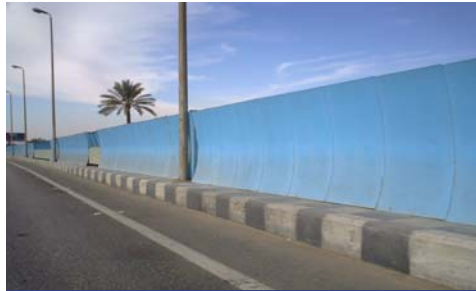
Picture (4-12) Noise Barrier at 26 th of July Corridor
