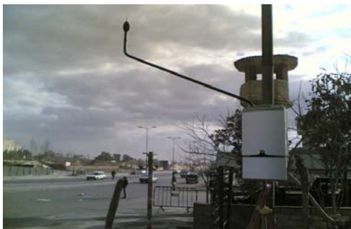
Picture (4-4) Tura Prison Station – Autostrad Road
