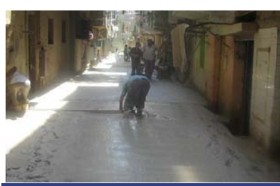
Picture (14-6) Paving roads with cement in Ezbet el-Walda
