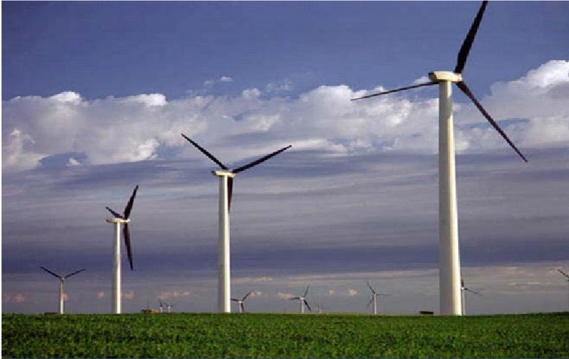
Pictrure (11-1) Wind Power station in Zaafrana
